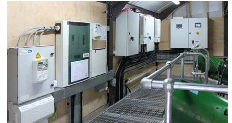
Electrical control room
